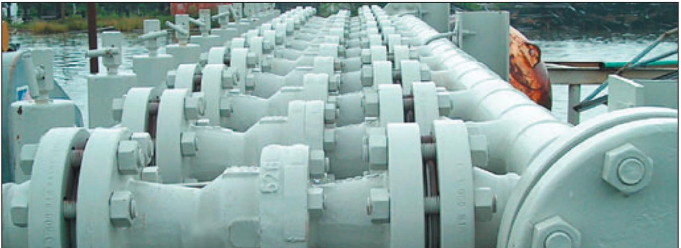
*PBV® Flanged Floating Ball Valves installed in a typical manifold application.*
