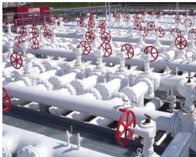
Contamination is avoided in multi-products manifolds.
